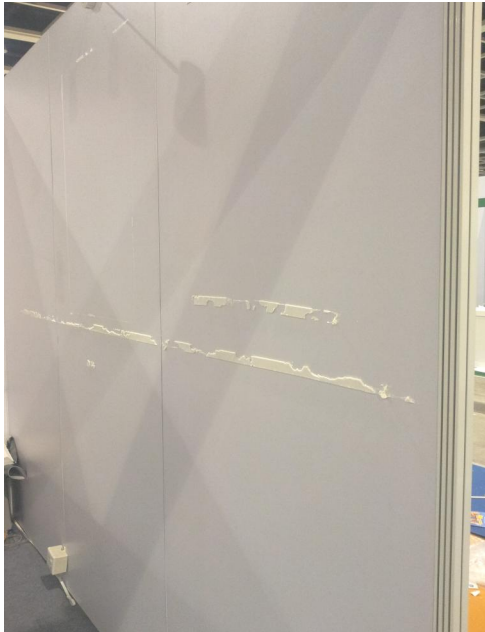
Double "Foam" Tape / lamination of low quality sticker directly onto panels
